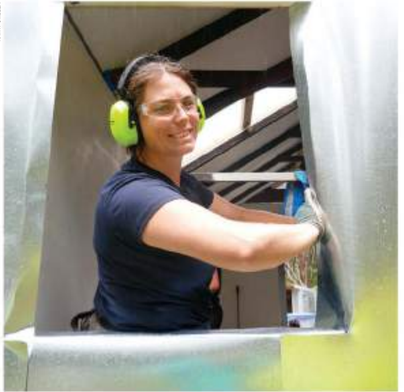
Helen Payn bends the iron cladding around the window frame
